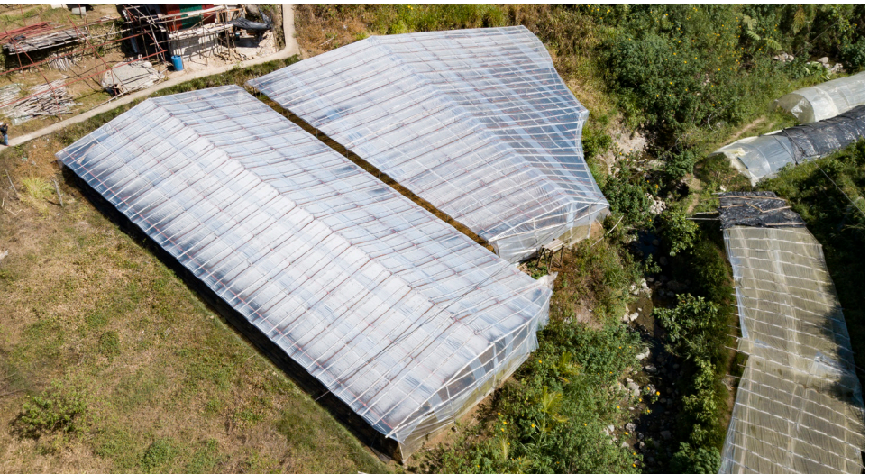
Fig. 3a. Aerial view of Chrysanthemum Greenhouse-type made of GI pipes in Bineng, La Trinidad, Benguet.
